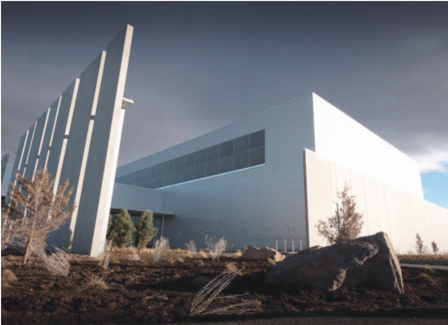
Ambient air flows through Facebook's data center in Prineville, OR, and cools the servers inside the 334,000-square-foot facility.
