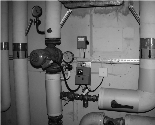
Figure 5. The control valve for the heating/ventilation system.
